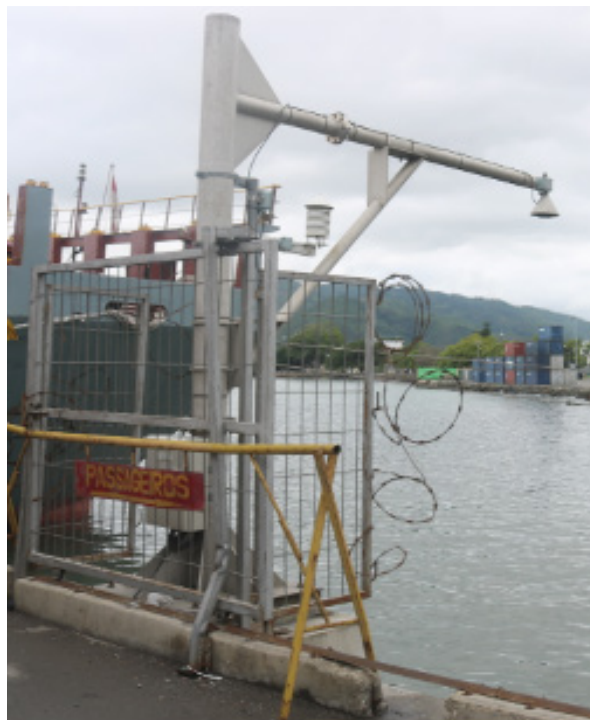
Fig. 1. Instalation of equipment consisting of an ultrasonic system and a control circuit at Dili Port (Timor Leste). Fotografer: Author (Abelito Filipe Belo), 20 January 2021
